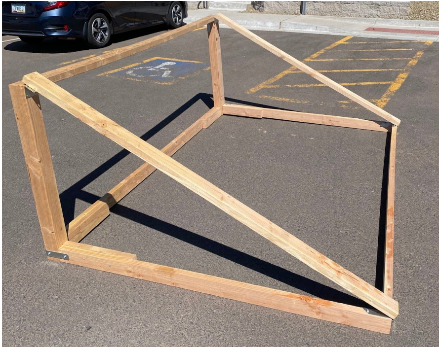
Figure 2: Completed mounting frame
