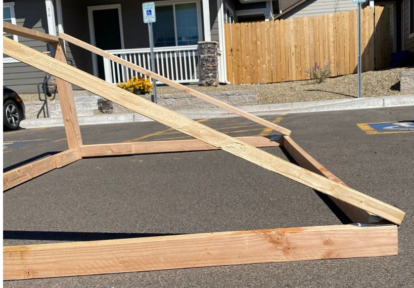
Figure 4: 30 degree angle joint and non-load-bearing 90 joint
